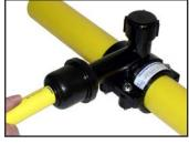
16 Verify that the O-ring is in the cap. Install cap on saddle hand tight. Do not use wrenches on cap.
